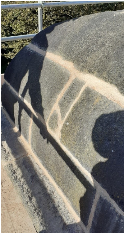
Top of bellcote repaired and repointed—repointing proceeding at lower levels.
