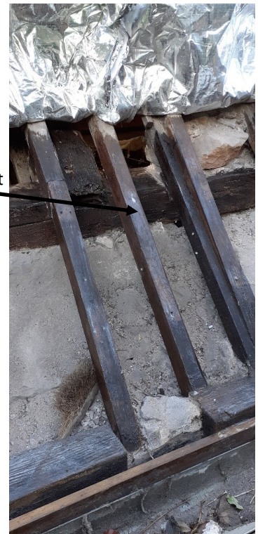
Wall head cleared of rubble infill
