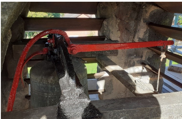
Bell frame / metalwork treated and painted to match existing
