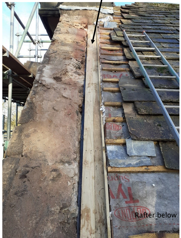
Secret gutter set out in relation to last rafter position (to gain maximum depth / upstand against copings)
