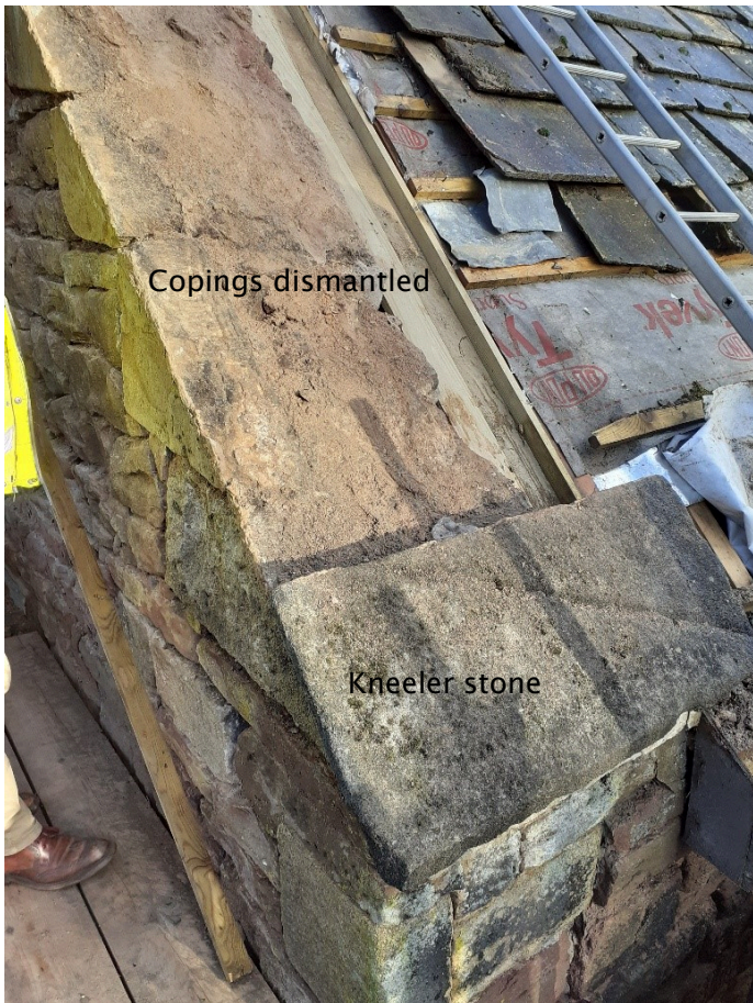
Construction of new secret gutter—at west end of south nave
