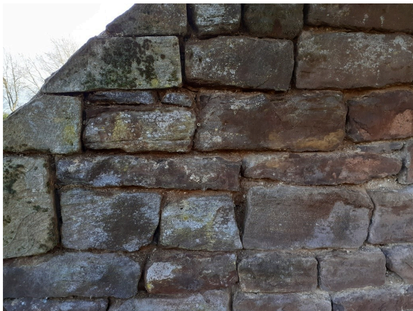
Raking out—west gable—prior to repointing
