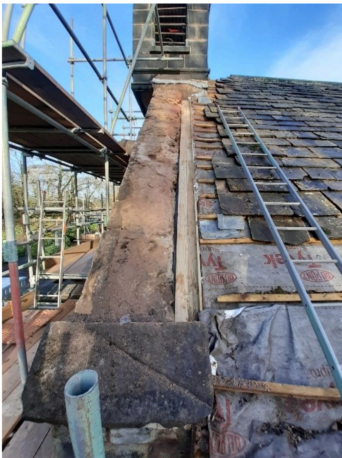
Construction of new secret gutter—at west end of south nave
