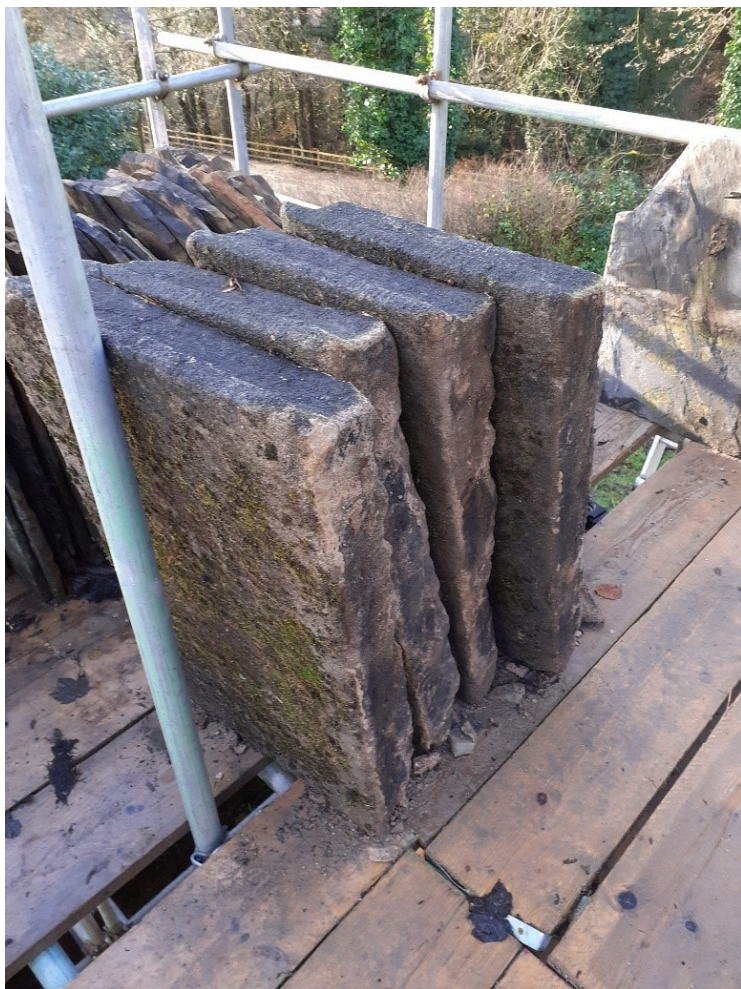
Coping stones dismantled prior to reinstatement
