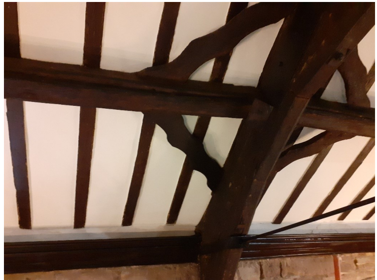
Ceiling panels painted. Timbers treated with Archdeacon's Mix.
