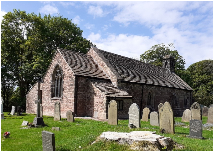
External repairs almost complete
