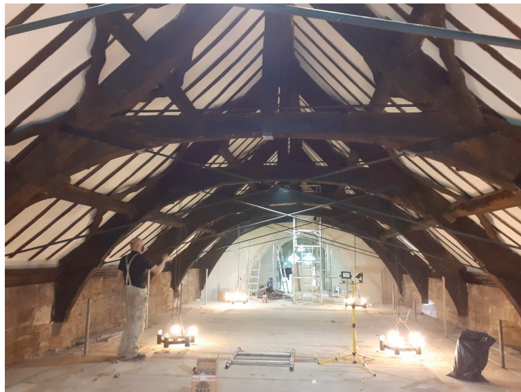
View looking east—decoration almost complete (except plastered walls).
